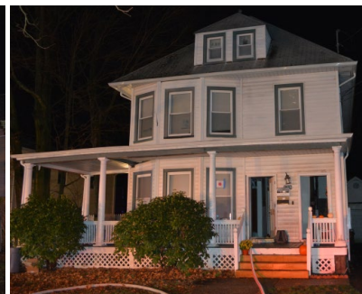
115 Washington Avenue Suffern, NY
